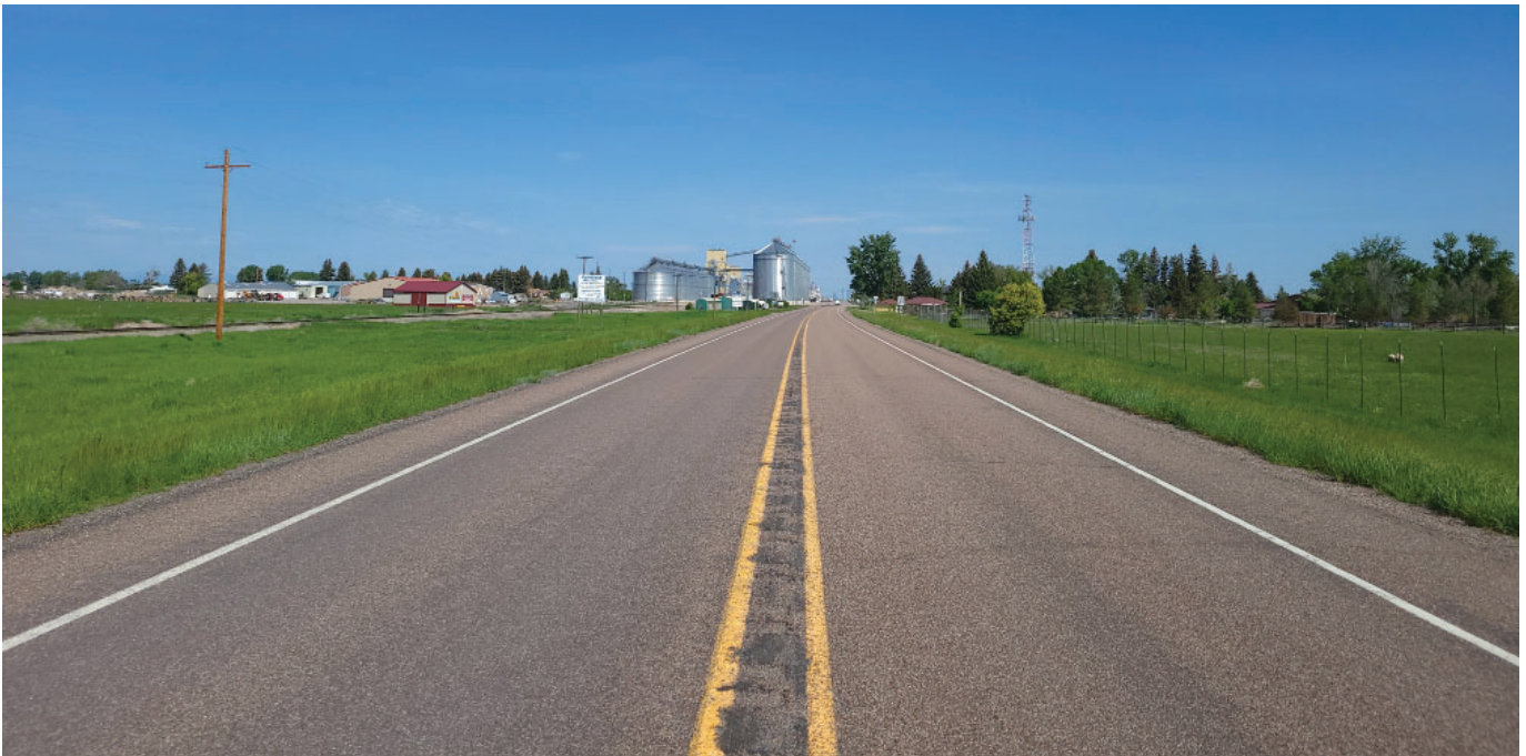
▲ Figure 1 - Outside of Fairfield
