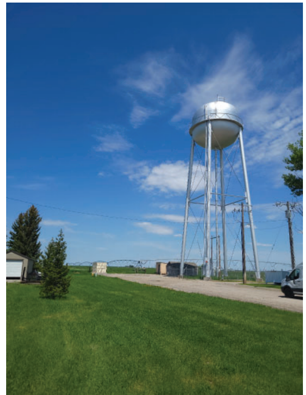
▲ Figure 4 - North Tank
